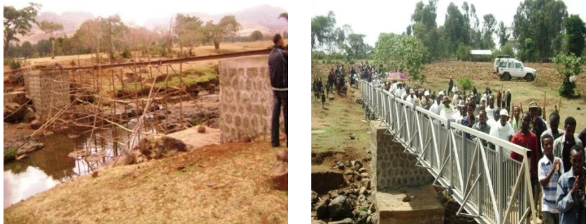
Figure 4.3. The bridge under construction and during the opening ceremony in 2009.
