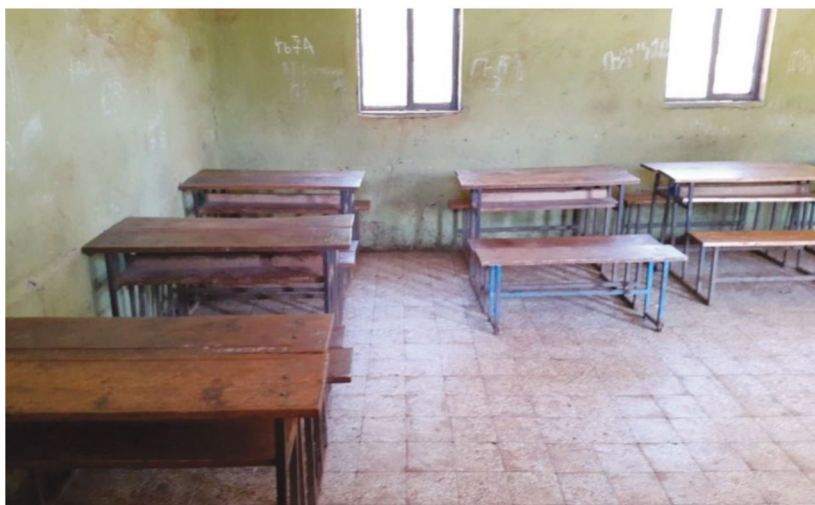
Figure 4.8. One of the elementary school classroom blocks (top) and a classroom (bottom) renovated in 2011 (photos taken in 2015).
