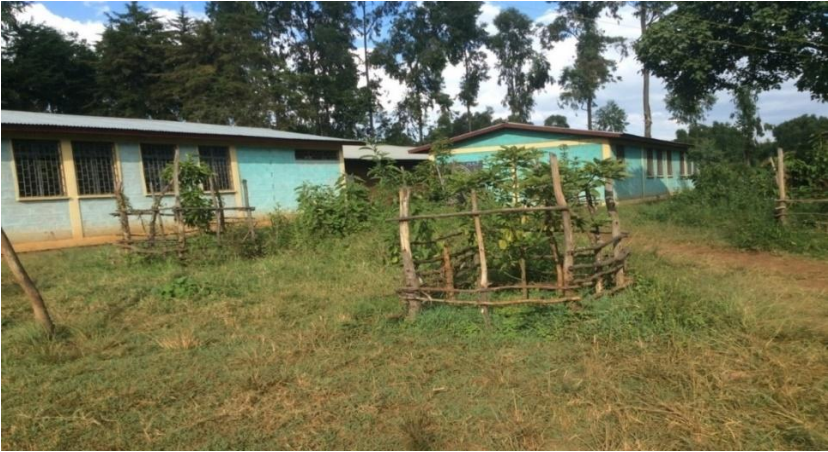
Figure 4.5. Two laboratory buildings constructed in 2010 (photo taken in November 2015).
